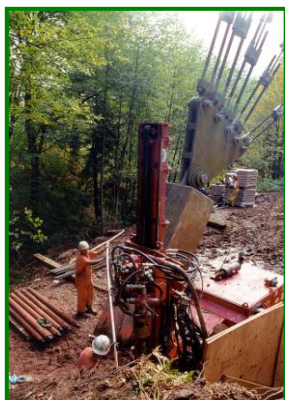
Compaction Grouting in Portland
