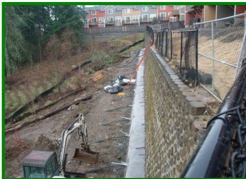
MSE Wall Remediation in Hillsboro
