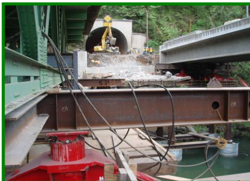
Rapid Bridge Replacement on OR-38
