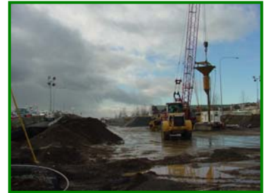
Stone Columns on SR-500
