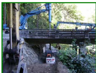
Drilled Shaft on OR-38
