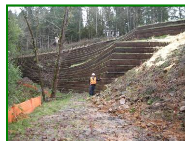
Reinforced Soil Slope on OR-38
